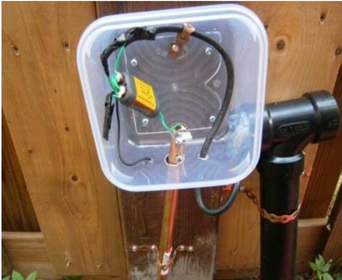
Picture 6 Transformer in the Plastic Food Box
