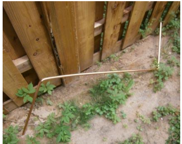
Picture 1 Pipe Prepared for Installation
