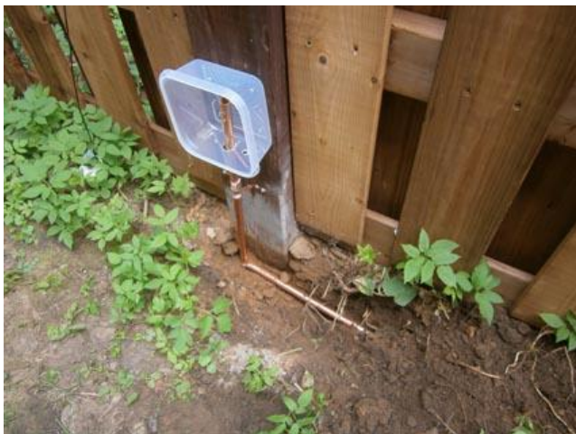
Picture 2 Pipe in Trench
