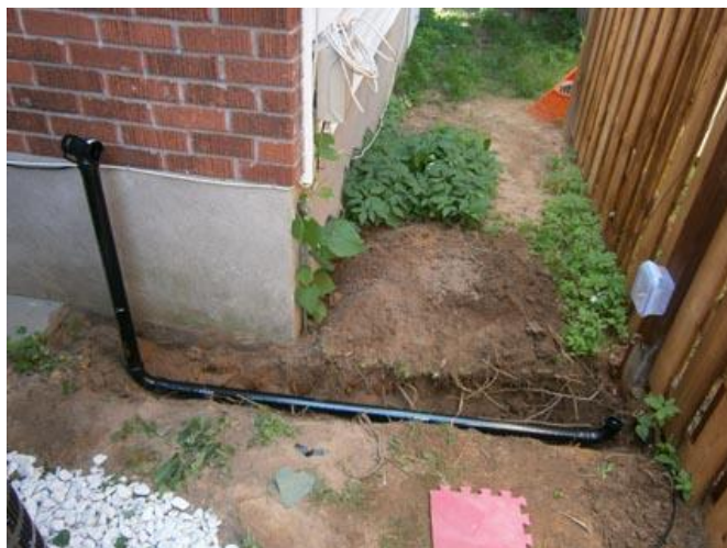
Picture 4 Trench with Plastic Tube
